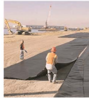
Below right: Placing the 15 foot wide rolls of Mirafi® HP570 geotextile
