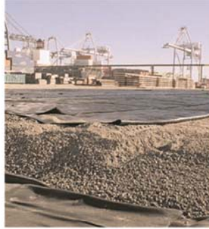
Below right: Placing the 15 foot wide rolls of Mirafi® HP570 geotextile
